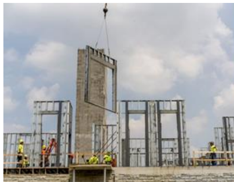
O-Zone New Construction
